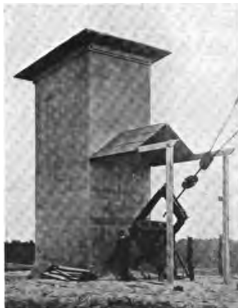
One of the Concrete Anchors to hold the Wireless Towers.
